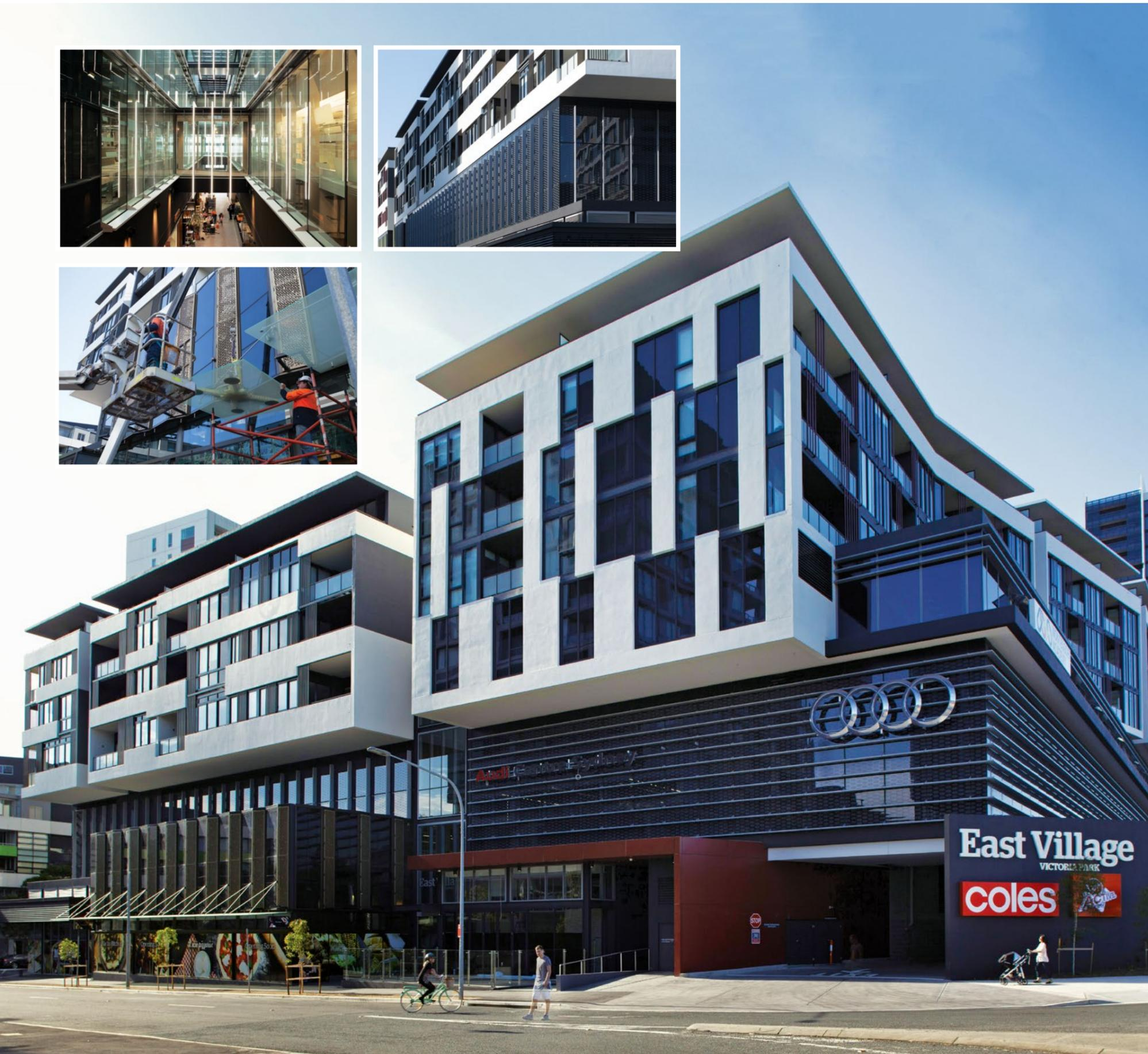
Undertaking the design, manufacture and installation of the aluminium and glass components on the East Village complex – including the development’s residential, retail and commercial aspects was AMA Aluminium + Glass Facades. This included aluminium and glass components for the external commercial curtain wall systems with horizontal and vertical fins, the internal atrium curtain wall over three floors and framed and frameless shopfronts both internally and externally.
